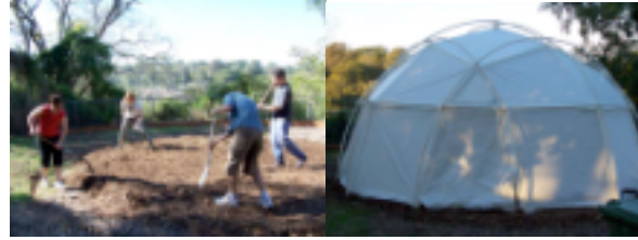
Figure 4. Mulch is leveled
